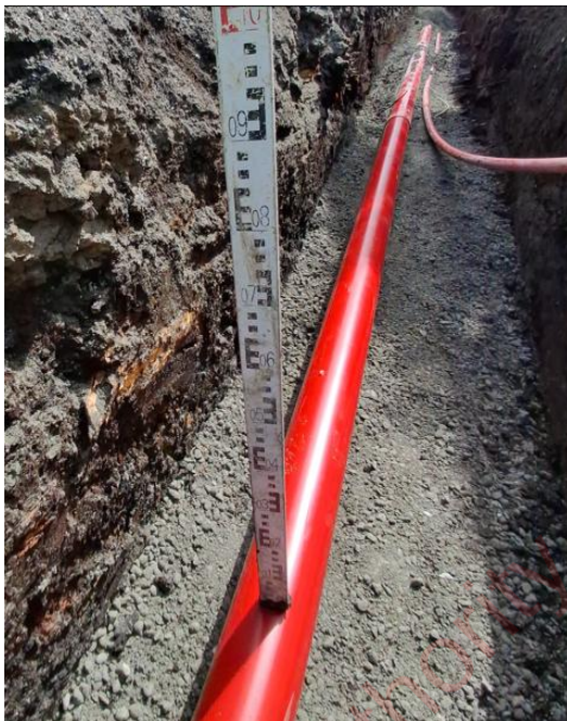
Plate 2-1 Typical Single Cable Trench View
