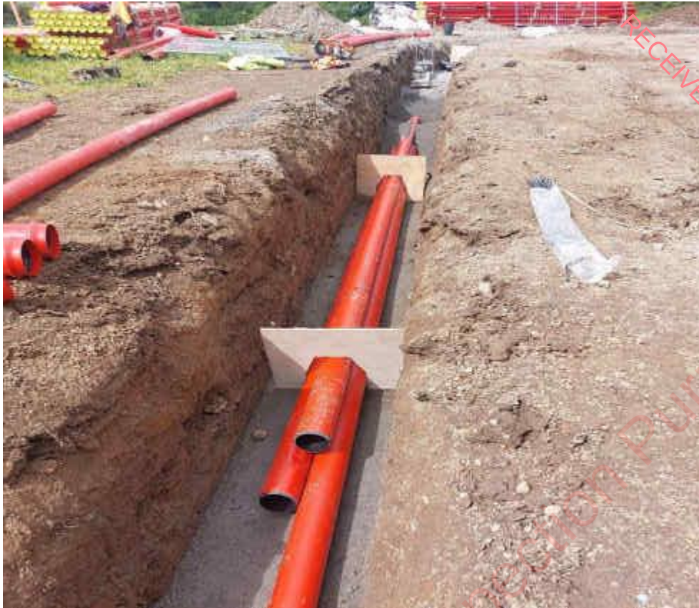
Plate 2-5 Typical 110kV underground duct installation on private land
