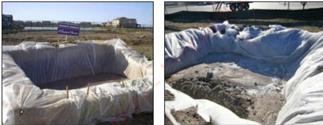
Plate 3-2 Typical concrete wash out areas
