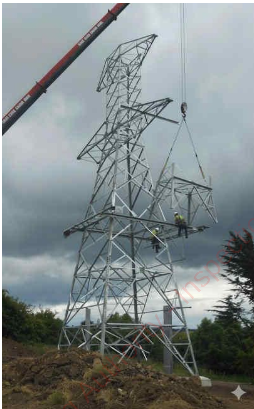
Plate 2-11 End Mast under construction
