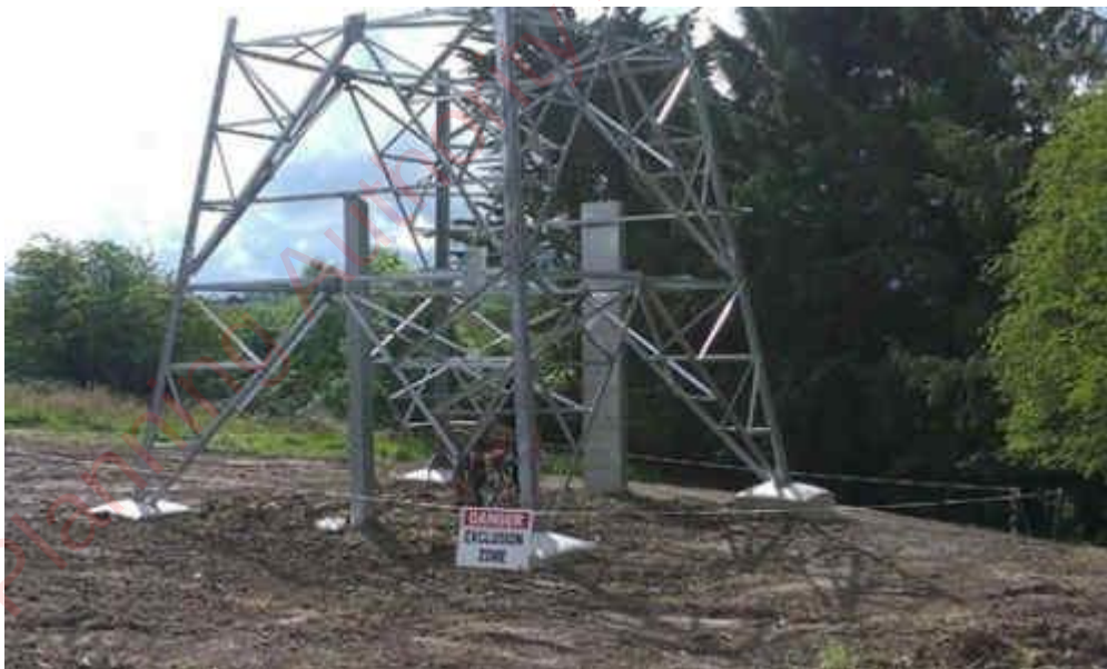
Plate 2-10 Base of end mast structure backfilled
